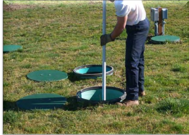
Septic tank inspection in process
