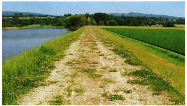
A levee protects adjacent farmland from flooding.
