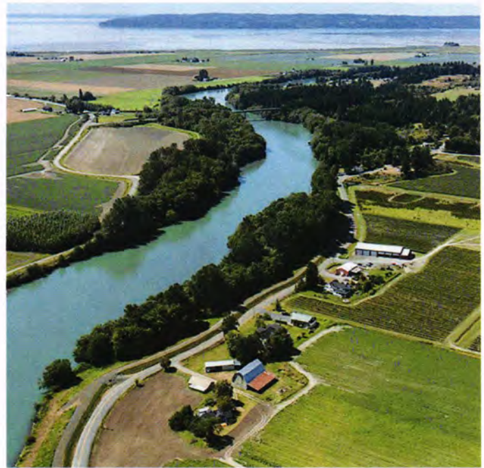
Levees and dikes protect Skagit farmland from flooding.
