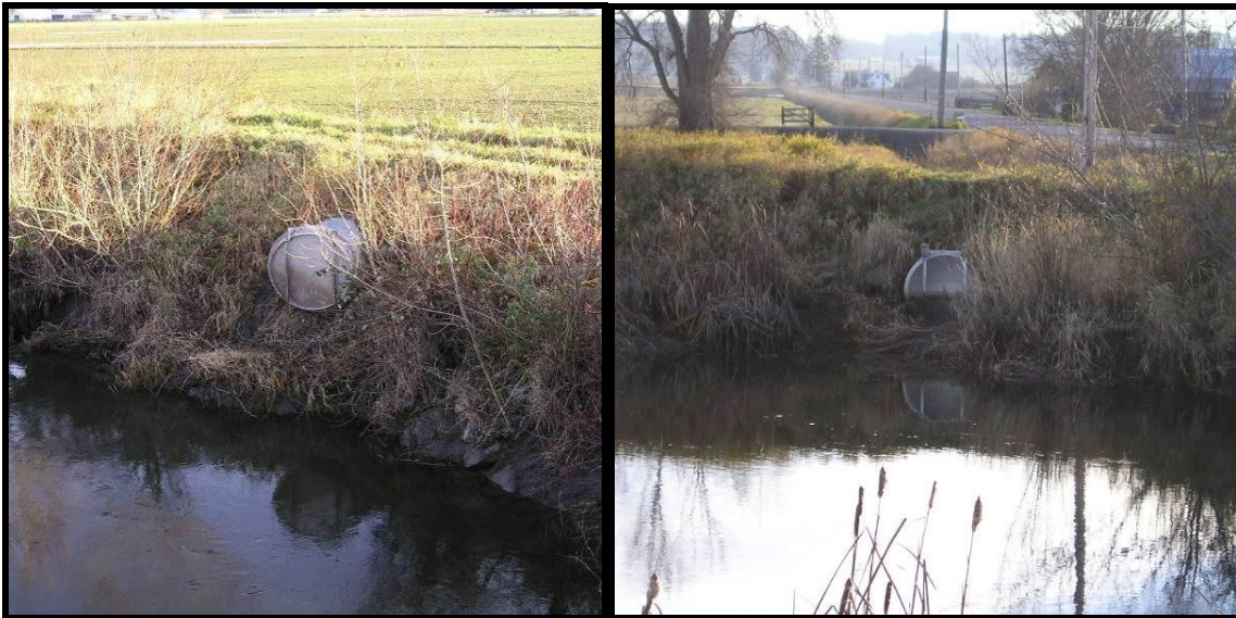
Figures 1-2 & 1-3 Floodgates, Drainage District 25 – Samish River system.
