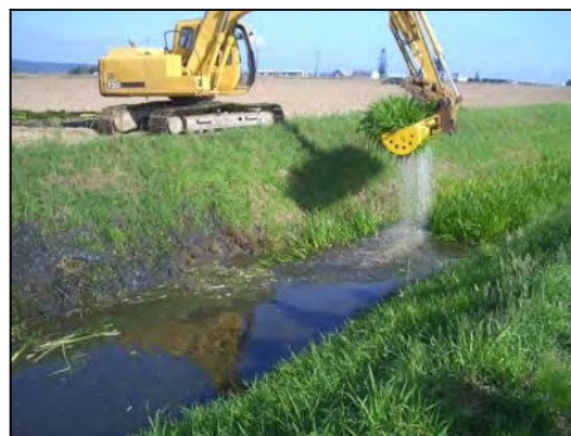
Exhibit 2-7. Ditch Cleaning with Mower Bucket
