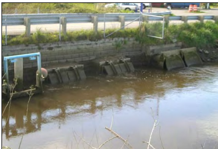
Exhibit 2-5. Tide Gates and Bridge on Edison Slough
